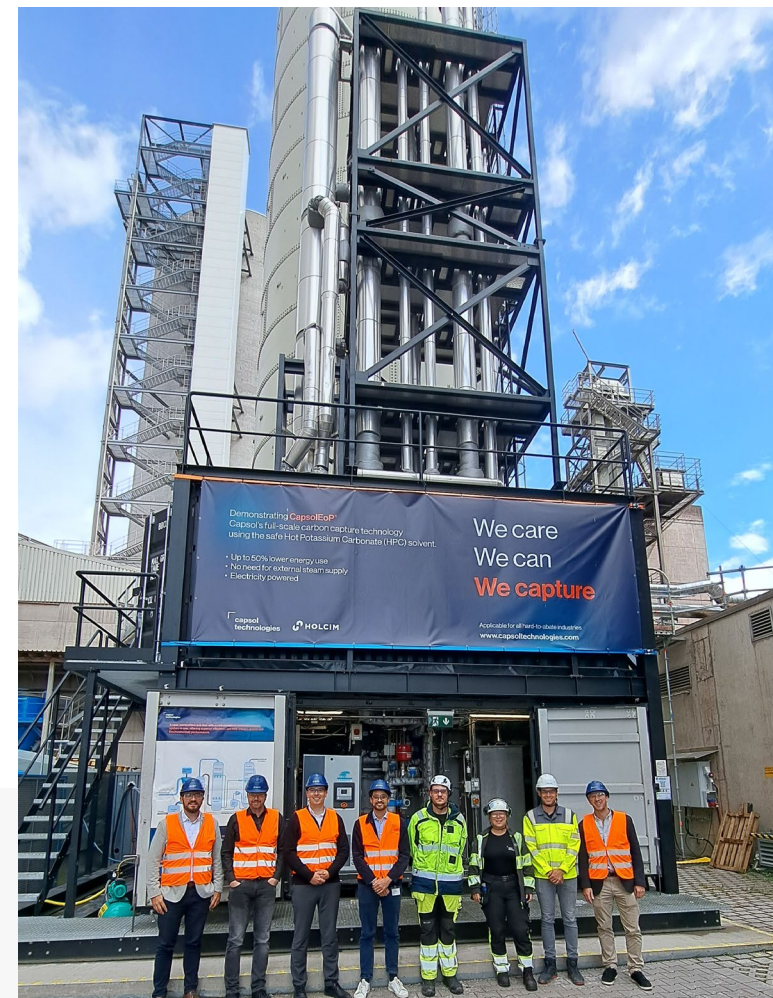
Finished campaign: Demonstration at Holcim Cement plant in Germany
