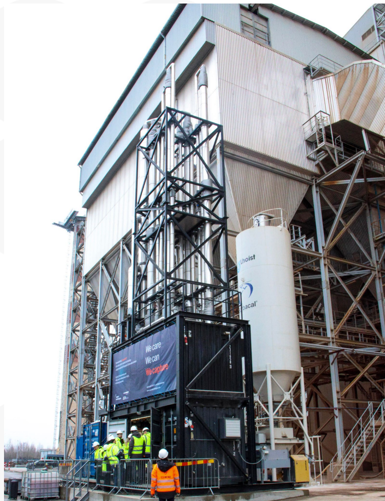
Baltic: Demonstrations with liquefaction at SCHWENK cement plants in Latvia/Lithuania
